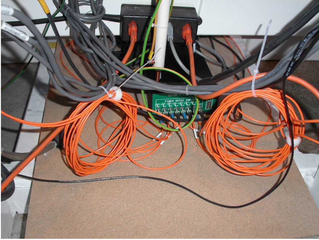
Figure 2: This box replace the previous TTL distribution box. It is located at the center of the kicker, on the lower frame. The visible front view shows the possible over-current trip LEDs. The non-visible back view has the TTL input signal, the four TTL output signals, towards each cabinet, and the TRIP monitor TTL signal as well as optical out for relay purpose.
